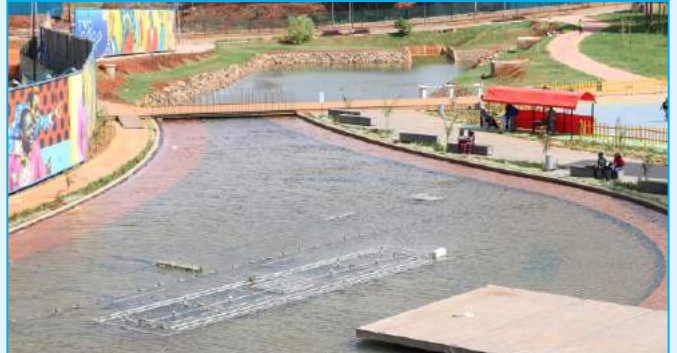
A view of the Two Rivers development water feature. All pumps, filters and controls were supplied by D&S.
