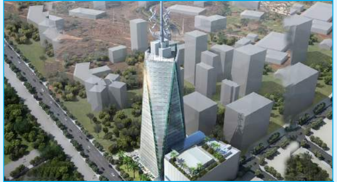
The impressive Britam Tower is set to become a landmark of the Nairobi skyline. All pumping equipment was supplied by D&S Westlands.
