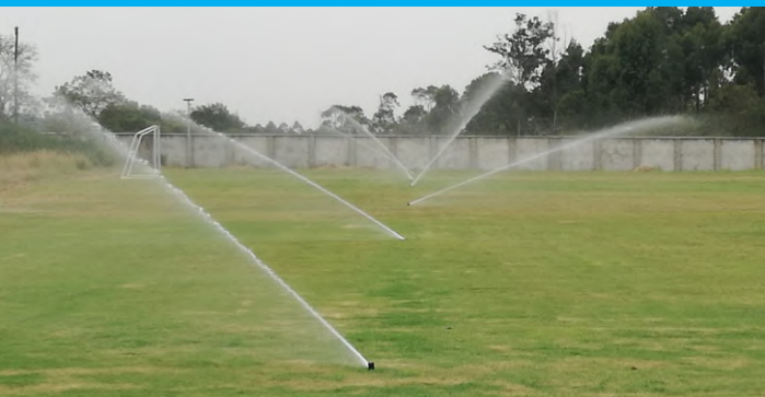
The newly installed smart irrigation system is pictured in action at the state of the art facility near Thika.
