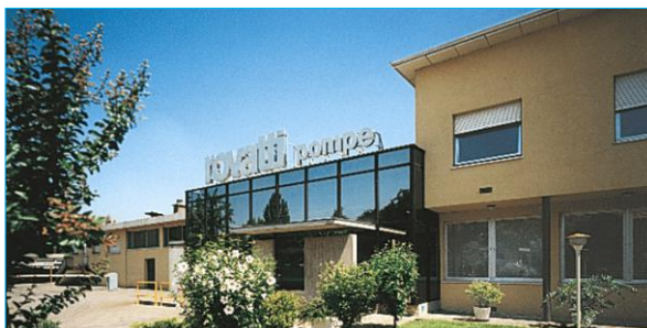
Rovatti Pompe Head Quarters in Reggio Emilia, one of several sites the company occupies.
