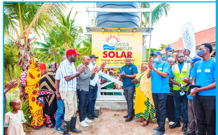
D&S Tanzania under MD Benjamin Munyao have supplied and installed a Dayliff Suntower with Sunflo solar water pumping system for a local community in Kigamboni. Pictured are staff led by the MD together with recipients during the commissioning of the project.
