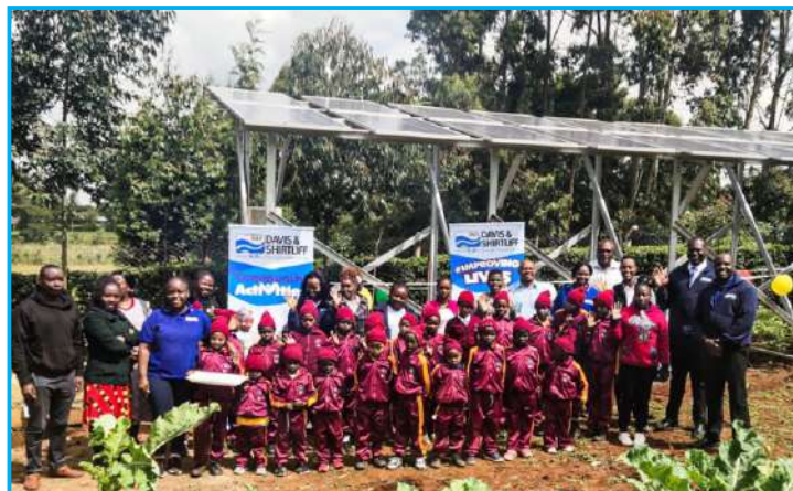
D&S HO #ImprovingLives Initiative have supplied and installed a Dayliff Solar pumping system to Save a Soul Children's Centre Limuru, a home to over 30 orphans and victims of abuse. Pictured during the handover ceremony are D&S team led by Solar Sales Manager Michael Njeru together with staff and children from the Centre.
