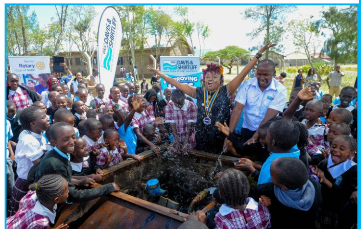
D&S Rongai under branch manager Amos Mutunga in partnership with Rotary Club of Nairobi Nabo have supplied and installed a Dayliff submersible motor at Ereteti Primary School to rehabilitate a damaged borehole. Pictured is Amos, Rotary's Wanjiku Wairia and students from Ereteti during the commissioning.
